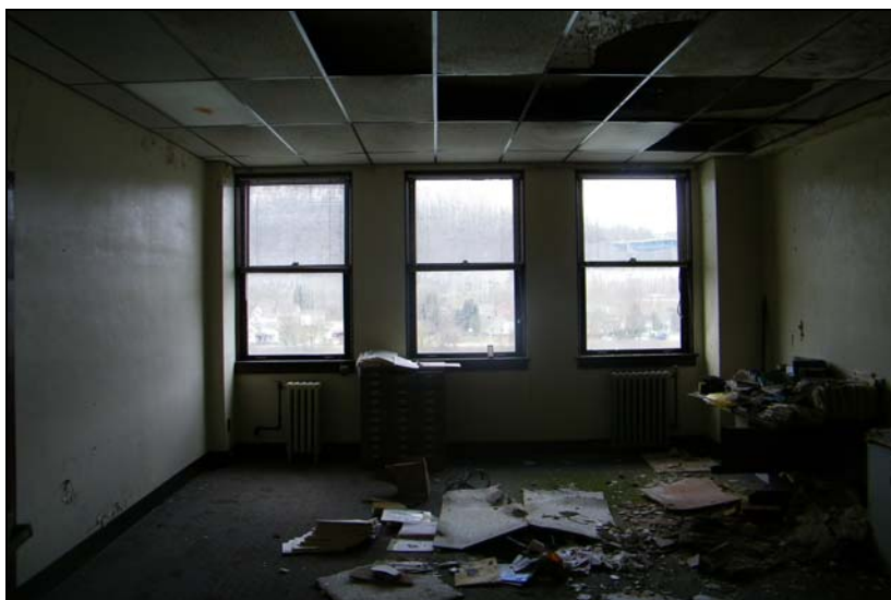
Typical Upper Floor with water damage.
